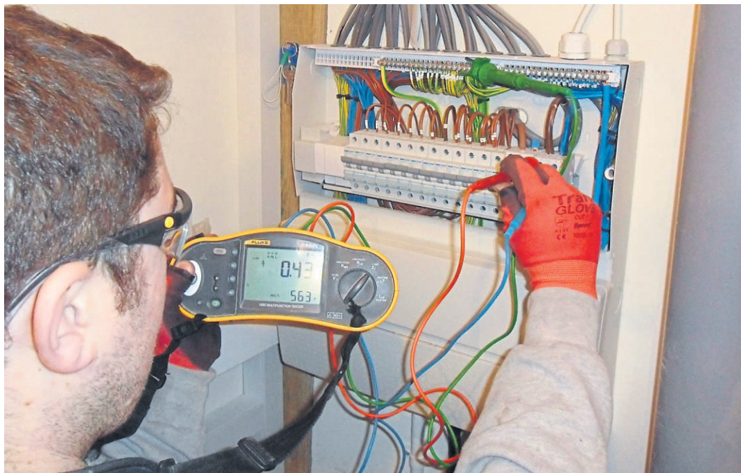
RGV electrician carrying out an installation test
