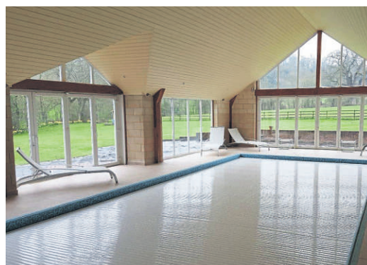
Swimming pool heated by RGV Panasonic ASHP
